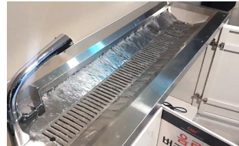
Trench-type drainage system
